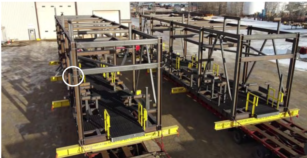
Figure 4.2: Pipe rack structure with an exterior beam-to-column connection highlighted (WF Steel and Crane 2021)
