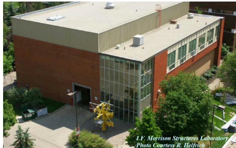
The IF Morrison Structures Lab at the University of Alberta Photo Courtesy R. Helfrich
