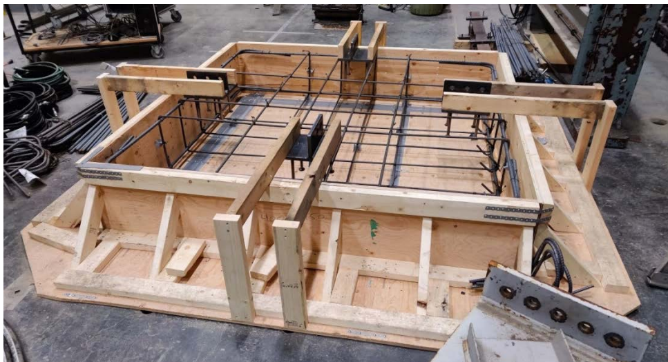
Figure D.4 Installation of SEP4 embedded plates
