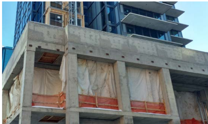
Figure 4.1 Embedded plates located close to the edge of a concrete beam
